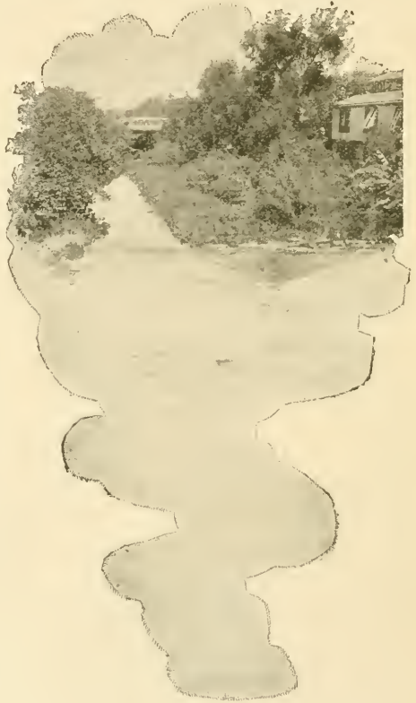
CROCKET STREET BRIDGE OVER SAN ANTONIO RIVER.
